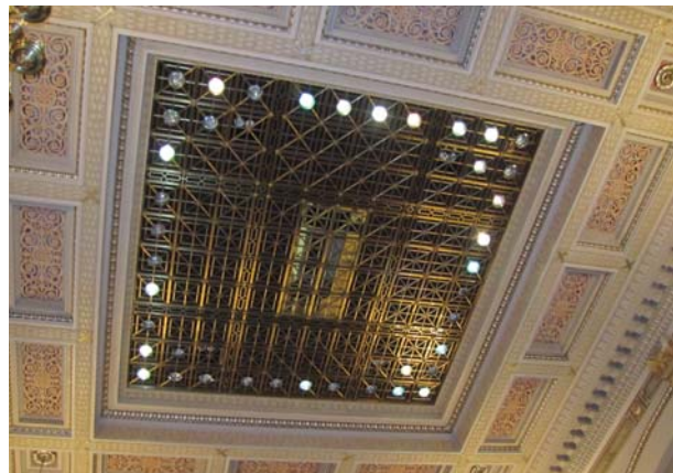
Figure 20: Senate ceiling laylight, showing downlight configuration
