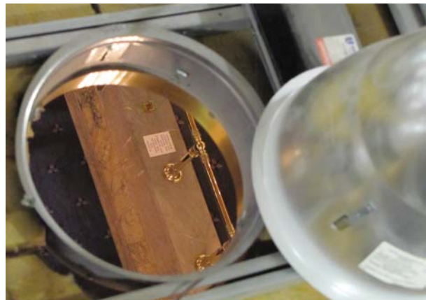
Figure 17: Metal ring added for larger light fixture
