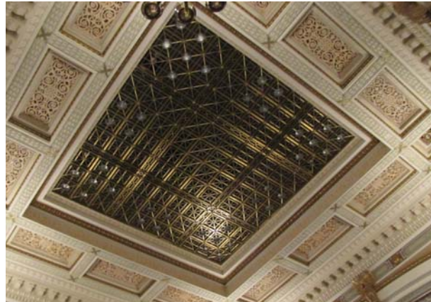
Figure 16: House bronze ceiling laylight
