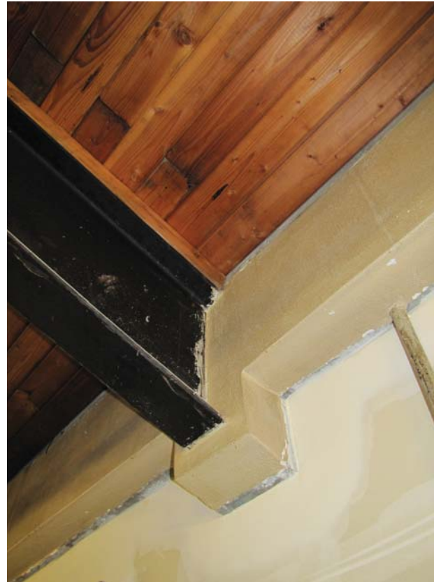
Figure 26: Wood decking above exposed steel beams.
