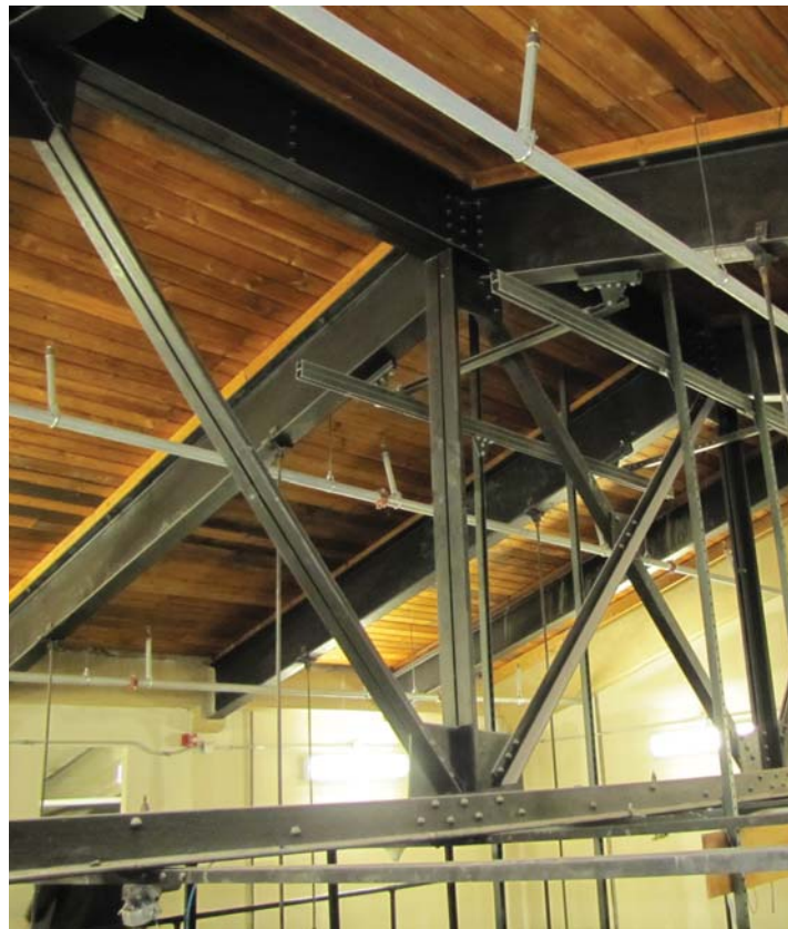
Figure ES07: Wood decking shown replaced the original skylights.
