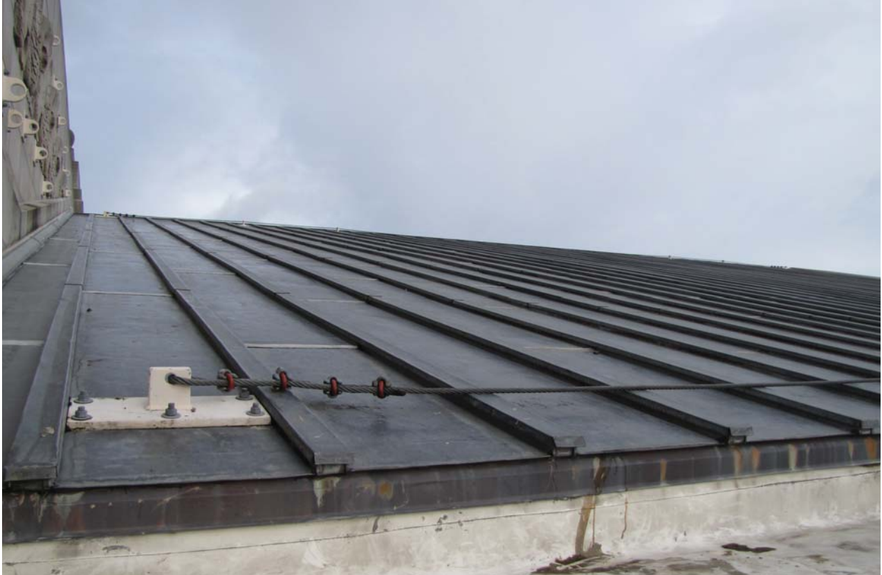
Figure 58: Existing roof at House and Senate Chambers
