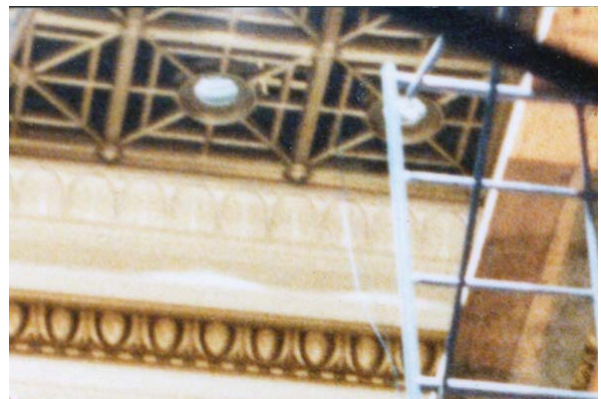
Figure 09: Light fixture at Chamber ceiling laylight, 1983 Courtesy of Washington State Archives.
